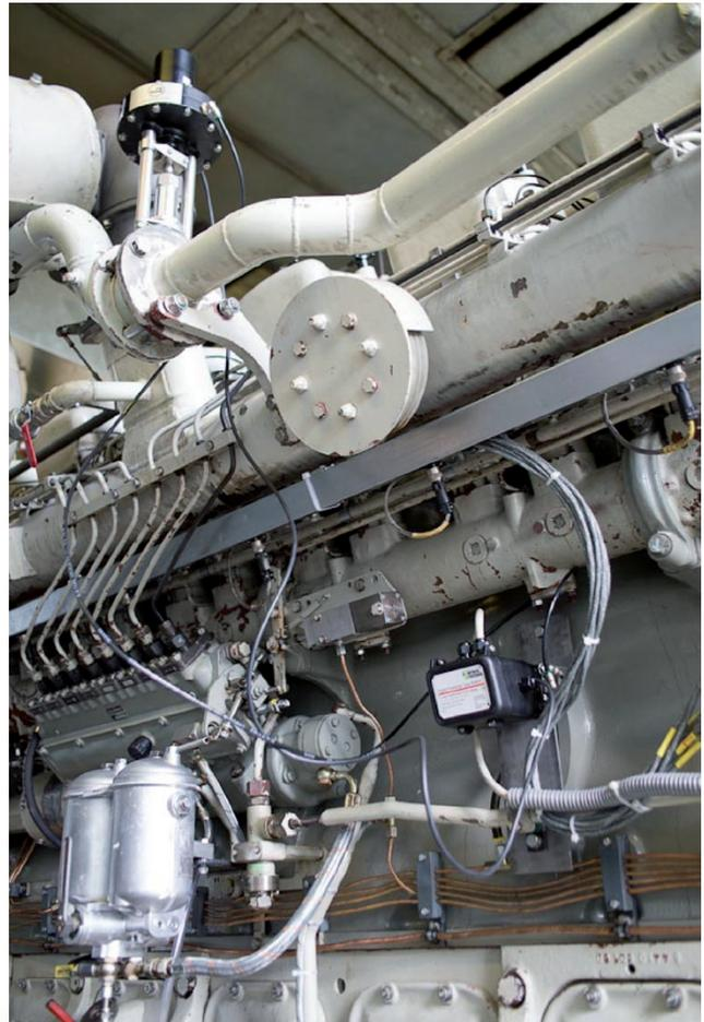
*One of the 1.58 MW power generators (MWM) at Munich Airport with Schubert & Salzer Control Systems' sliding gate valve (upper left) and, lower right, the digital positioner which is mounted separately to protect it from vibration.*
